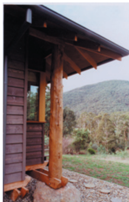
Suitable window thickness and window protection, combined with closure of eaves and keeping shrubs and trees well away from the residence, will help minimise the susceptibility of a house to bushfire attack. (Photo courtesy of Paul Harr, architect.)
